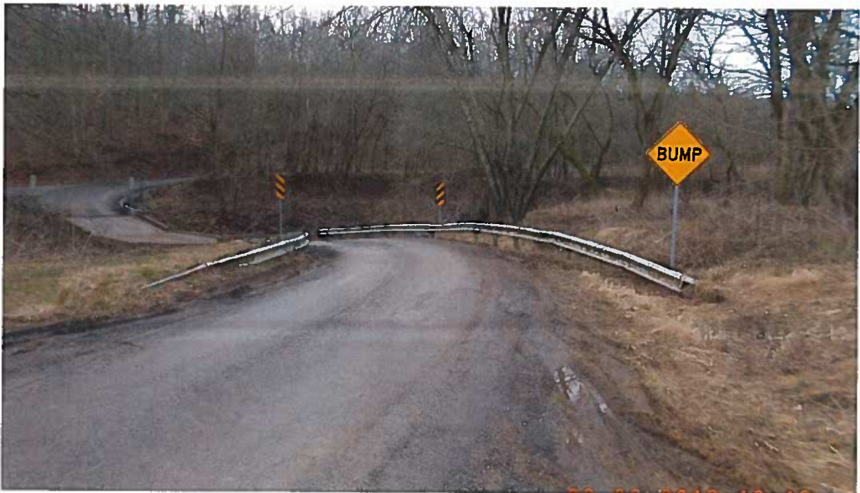
Approach - Looking Back Station
