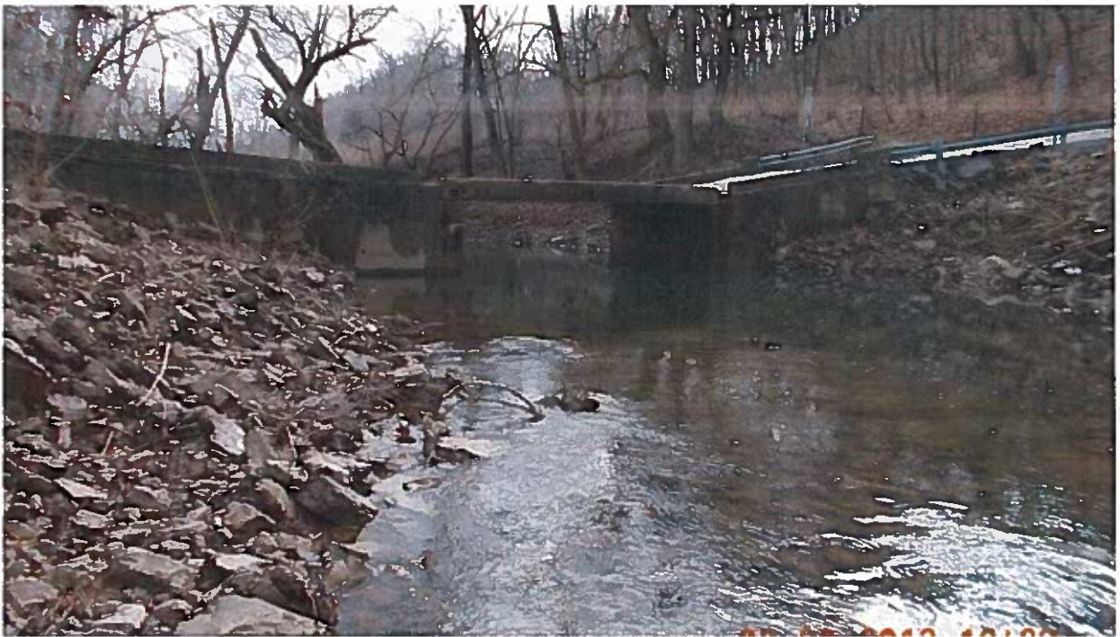
Elevation - Looking East
